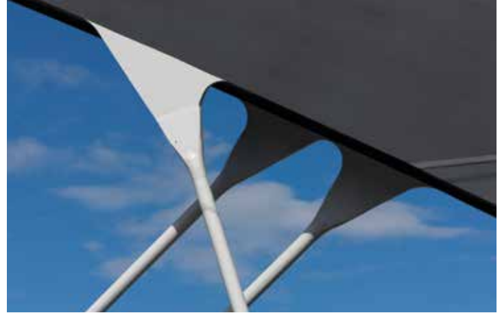
Upset-forged hanger connection
