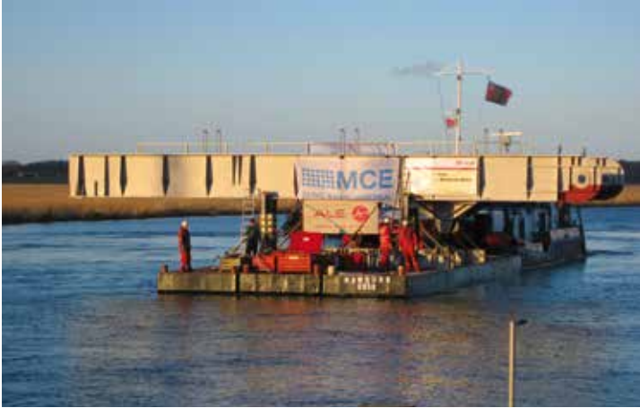
Floating of the bascule bridge
