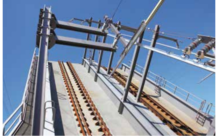
Lifted bascule bridge
