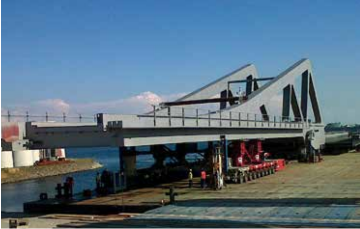
Loading of the road bridge in Wilhelmshaven
